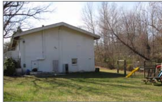
Back view of church bldg
