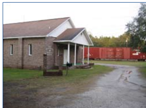
Front view of building
