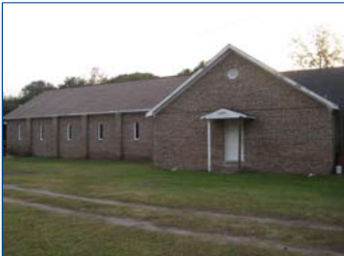
Side view of building
