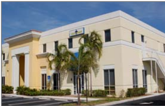
Front view of building
