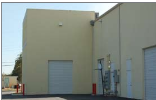
Back view of building
