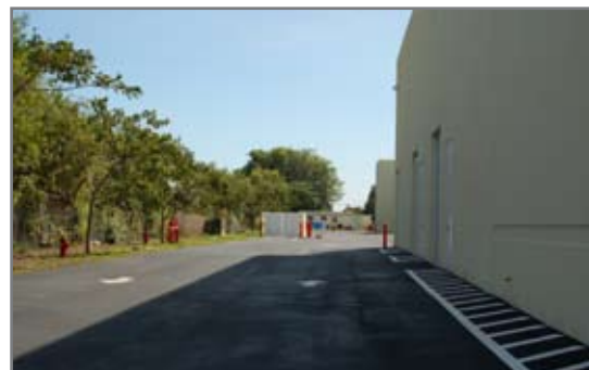
Back view of building
